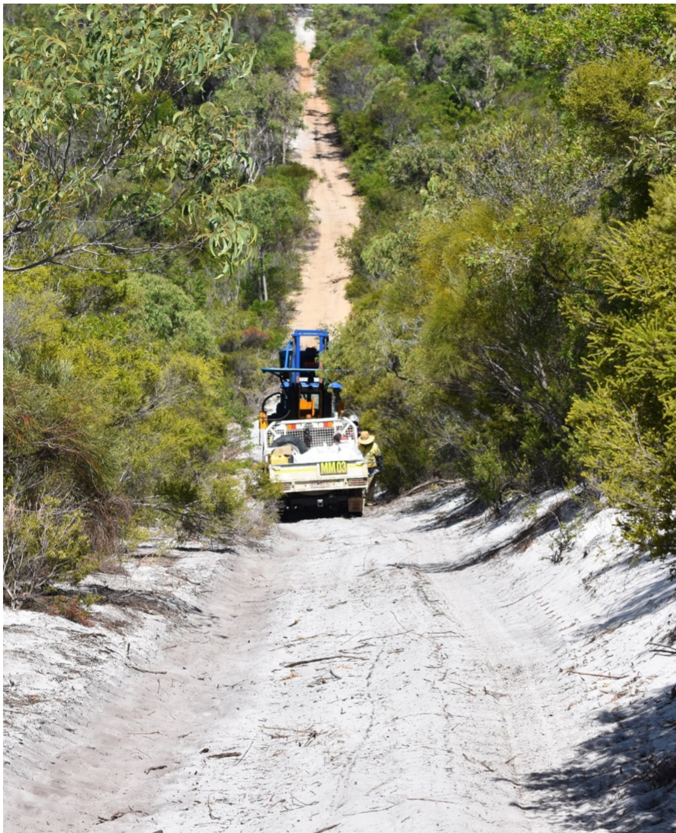
Figure 2: Photo of Yearlong Contractors vacuum-based drill rig working at CFS project
